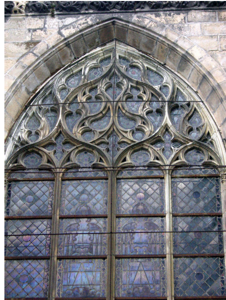
Limoges Cathedral - Flamboyant Arch
